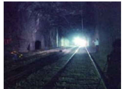
Blainville Line Electrification
