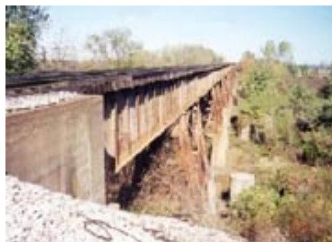
Ohio River Bridge Steel Repairs, Cairo Subdivision - Mile 363.40
