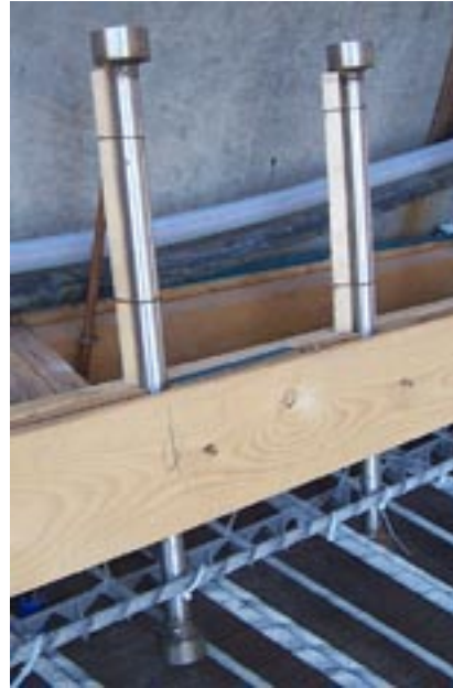
Red River Bridge: Stainless Steel Studded Anchors for Traffic Barriers
